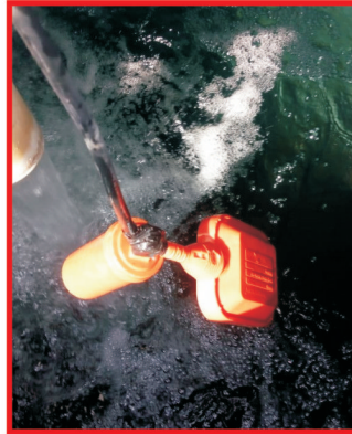
LEVEL CONTROLLERS AT OHT and STORM WATER COLLECTION PIT
