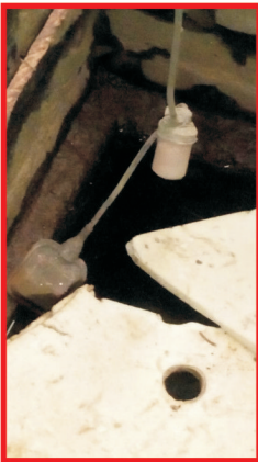
LEVEL CONTROLLERS AT OHT and STORM WATER COLLECTION PIT
