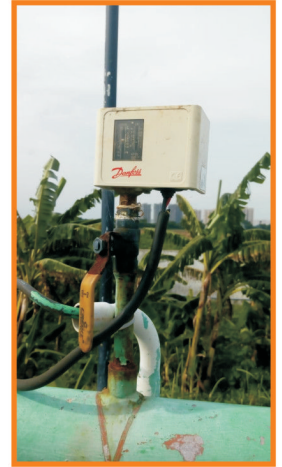
DIFFERENTIAL PRESSURE SWITCH AT STP
