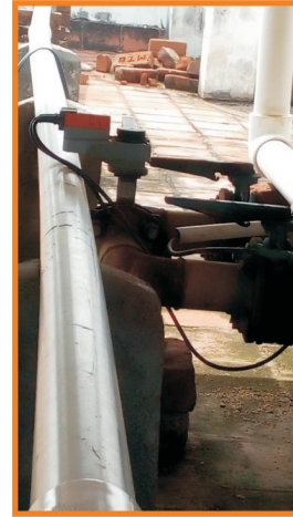
DIFFERENTIAL PRESSURE SWITCH AT STP
