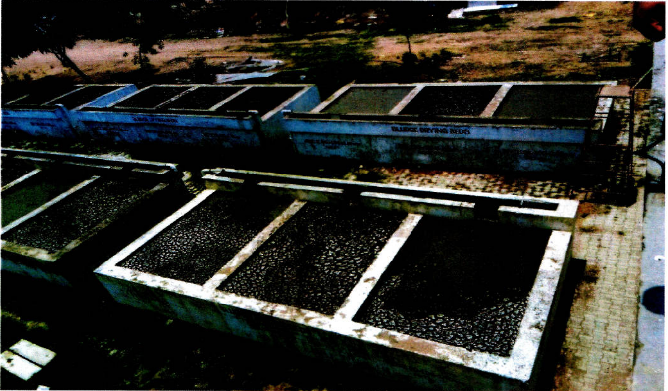
Fig5:sludge drying beds
