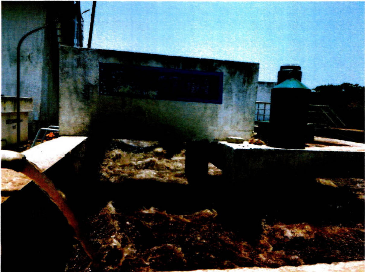
Fig3:aeration tank
